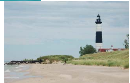
Big sable point lighthouse
